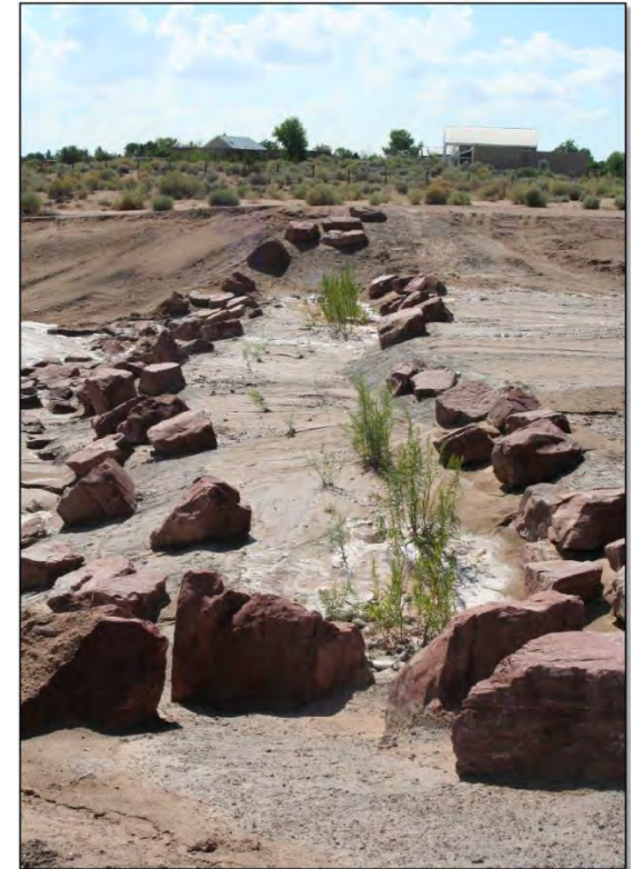
Photograph: Grade control structure in the Lower Montoyas arroyo incorporating planting strip. (Source: SSCAFCA)
