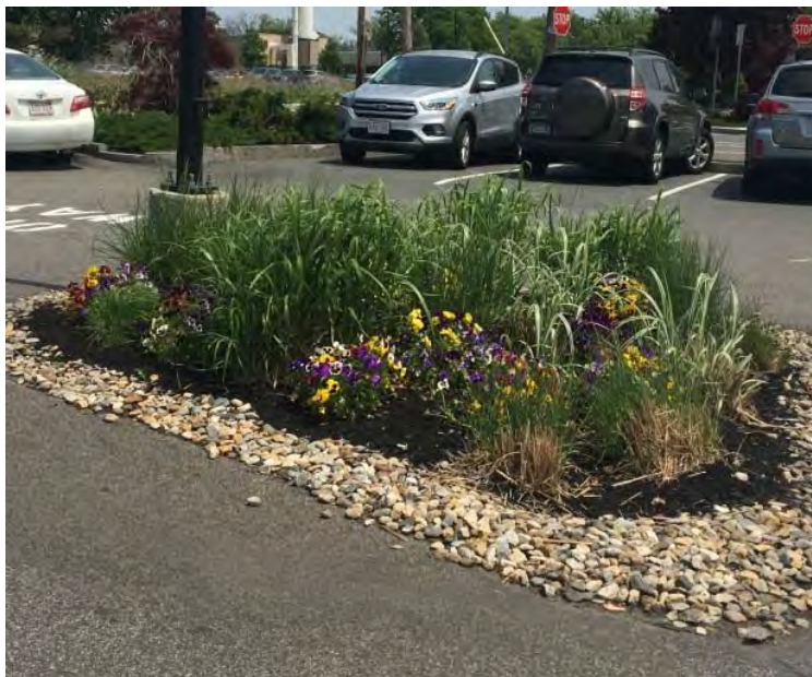
Example of Removal of Impervious Surface (1)
