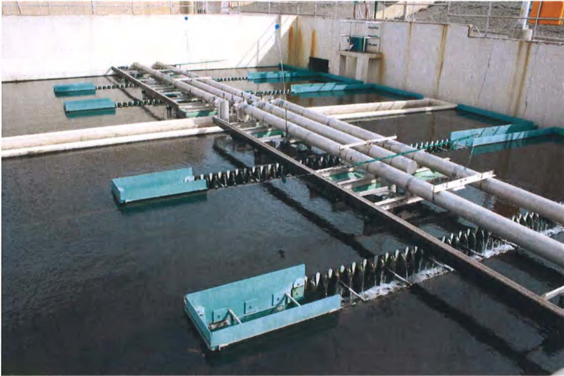
Figure 5: Secondary Clarifier Weirs and Clarivacs
