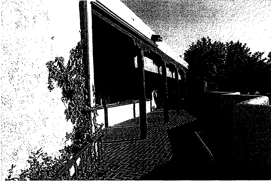
WEST ENTRANCE PORTAL, WOOD BEAMS ARE COMPOSITE WITH 2X FACING
