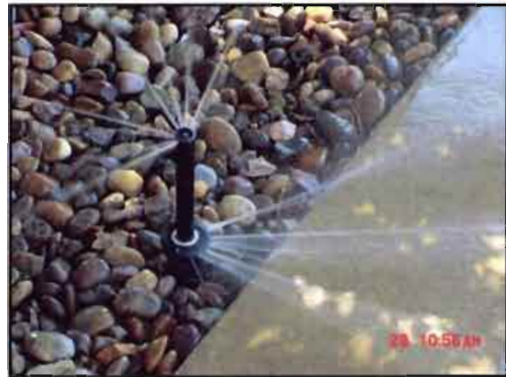
Figure 2-1: Sprinkler Leak
