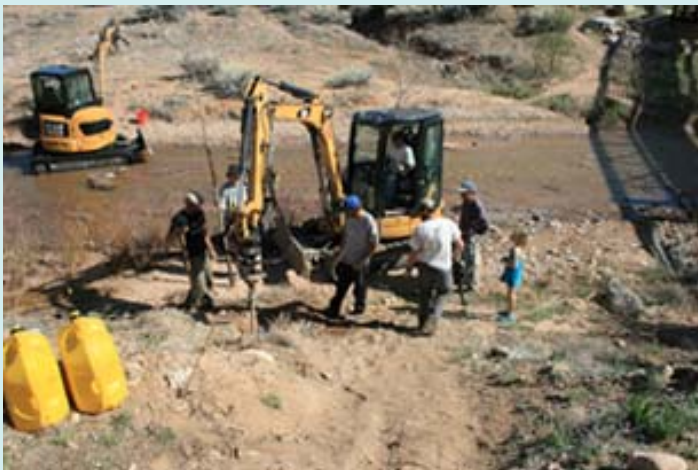
Native plants being planted along the Santa Fe River for restoration
