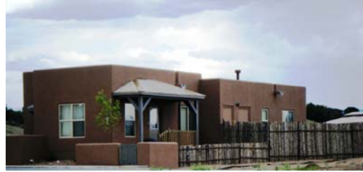
YouthWorks, Santa Fe Area Homebuilders Association and Santa Fe Habitat for Humanity for building an affordable green home using at-risk youth
