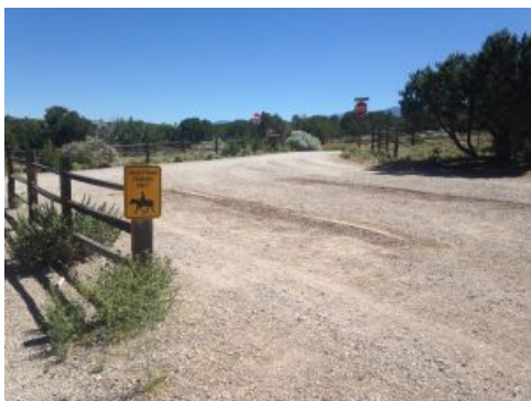
Finished product: over time, gravel around the wooden delineators is expected to subside about 1/2 inch to an inch.
