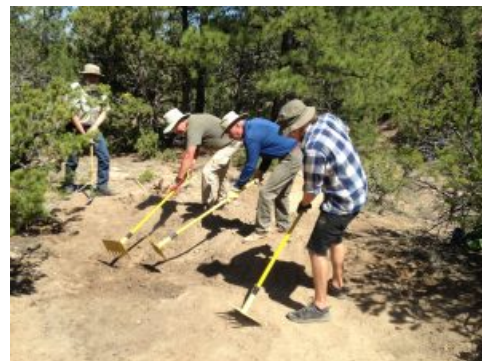
(2) Helping clear the drainage channel while building up dirt to pack on top of the rocks
