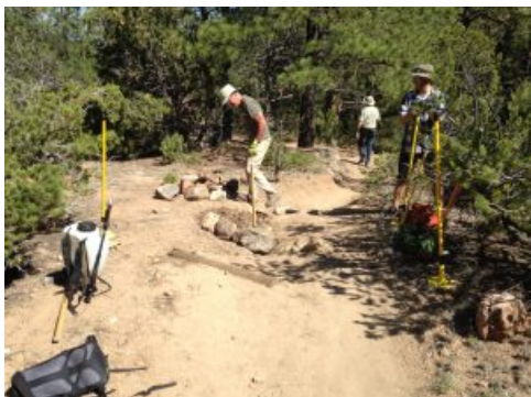
(1) Building a rock base to a new grade reversal; failing water bar in foreground
