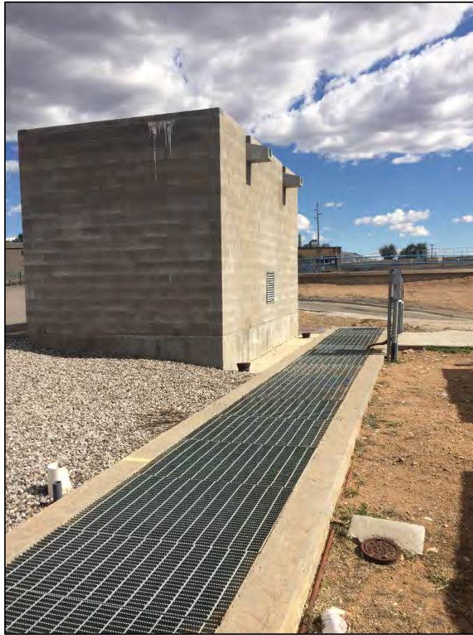
Reclaimed water is conveyed to multiple non-potable reuse sites from a series of pump houses along the effluent channel at the Paseo Real WRF.
