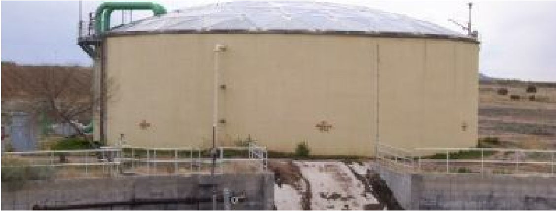
Sludge Storage Tanks - After the biosolids have been treated, the City's Wastewater Treatment Facility has the capability to store its' biosolids before disposing of them, either to the Sludge Injection Field or the Compost Dewatering Facility.
