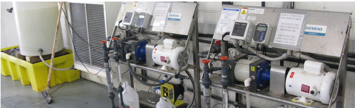
Polymer Pumps that add polymer to help in thickening the biosolids.
