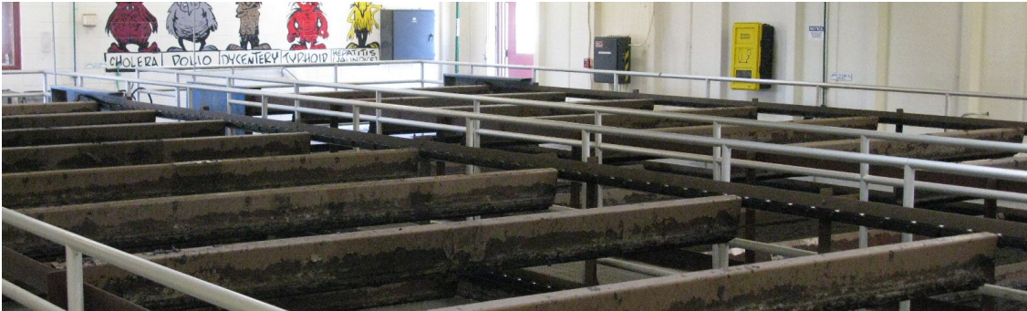
There are three separate DAF unit. Each unit has a 32,300-gallon DAF (Dissolved Air Flotation) tank with its own individual equipment apparatus so it can operate independently for operational flexibility. Two of the DAF Units are located side by side in one building. The third DAF Unit was added in 2009 for additional solids loading and to provide equipment redundancy and is located in a separate building.
