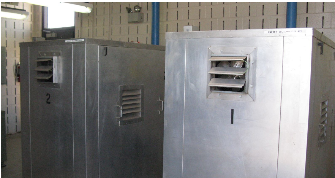
Grit Blowers enclosed in sound reducing panels.
