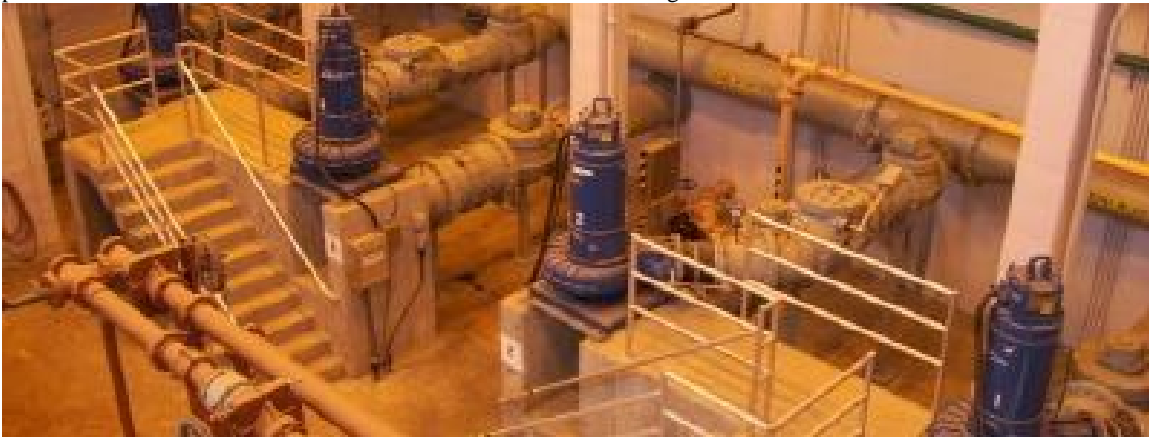
The wastewater from the wet wells is pumped by one or two of four influent pumps to the grit tanks.
