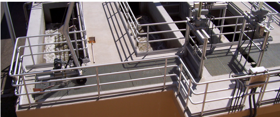
The wastewater flows through one of two grit tanks and is aerated.
