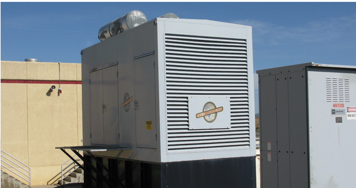
Generator by the DAF Buildings supply power to the DAF, Digester and Hoffman Blower Buildings. It also provides power to the Aeration Basin Mixers and the Secondary Clarivacs.
