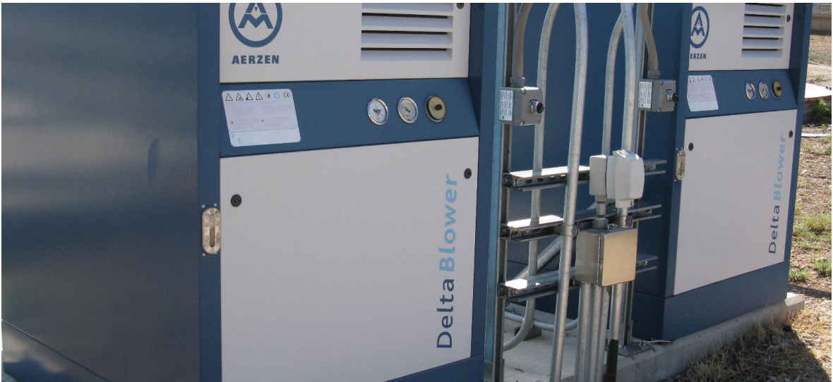
Two Aercen Delta air blowers provide air to the Post Aeration Basin where the effluent flows through to ensure permit compliance for dissolved oxygen. The blowers are alternated and run 24 hours each day.
