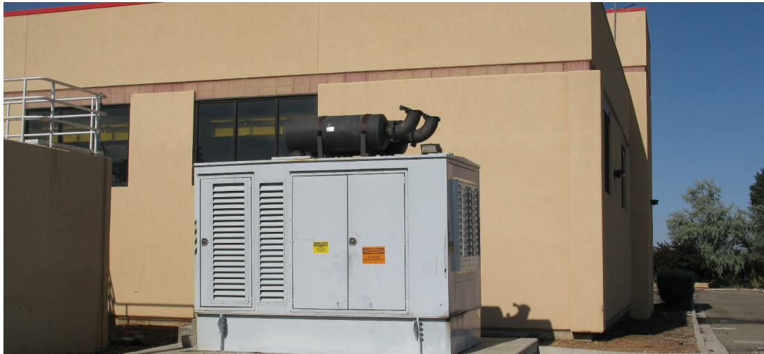
Generator by the Head Works Building supplies power to the equipment in the in the building, the Grit Blowers and the Primary Clarifiers.
