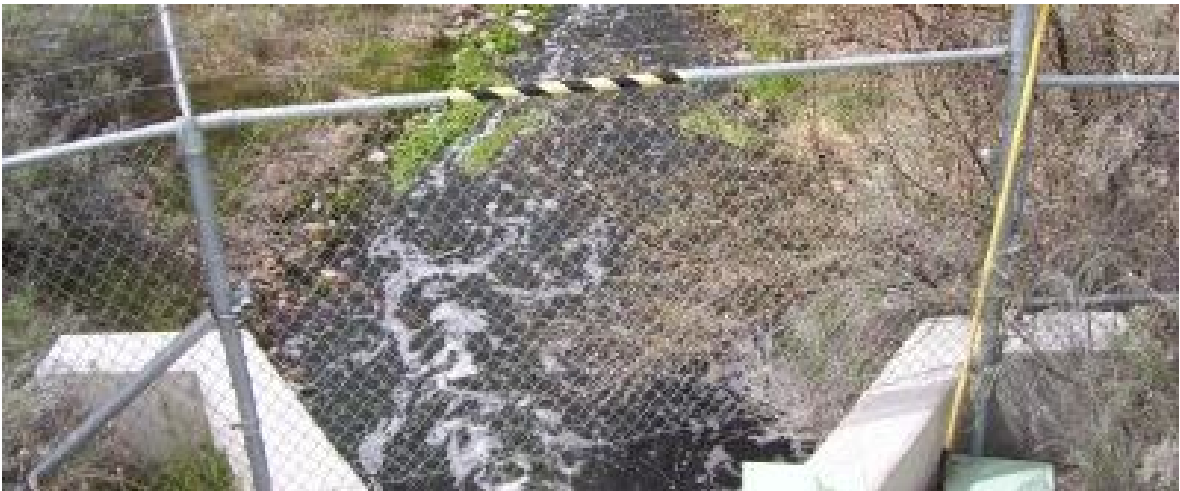
The plant effluent flows through the parshall flume where it is metered before leaving the plant and making its way to the Santa Fe River.
