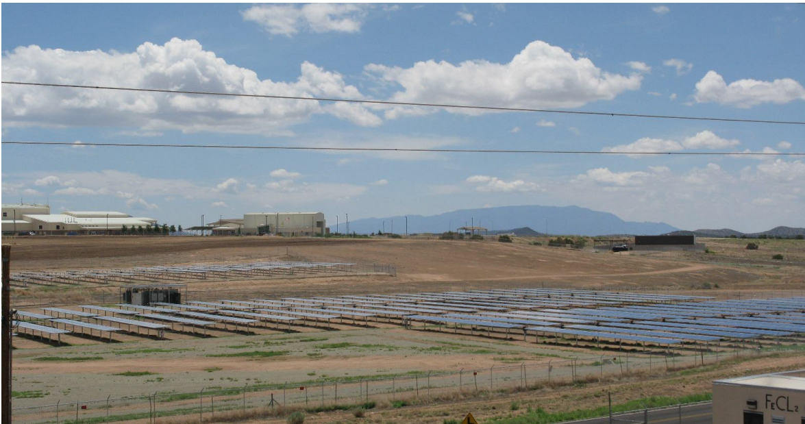
The City of Santa Fe has two separate Solar Array installation. These installations provide about one third of the Wastewater Treatment Facility power. The other two thirds power come from PNM. The solar panels shown above rotate following the sun during the day.
