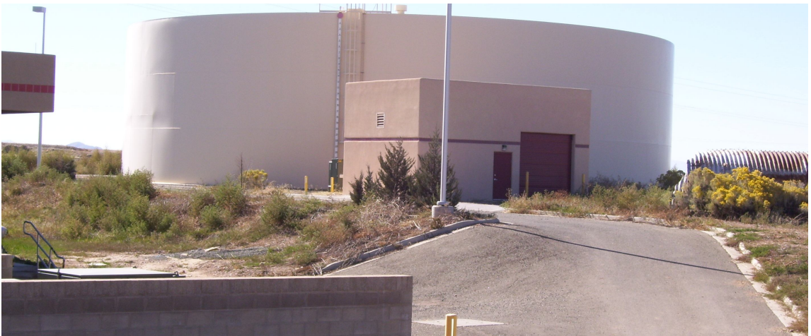
The non-potable reuse pump houses pump the filtered/disinfected non-potable water to various golf courses and sports fields.
