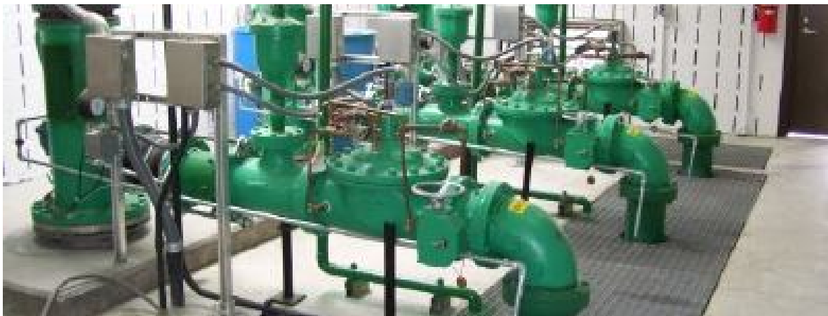
The non-potable water pump(s) system draws filtered disinfected water from the effluent channel to supply clean water for reuse as seal water for various pieces of equipment.
