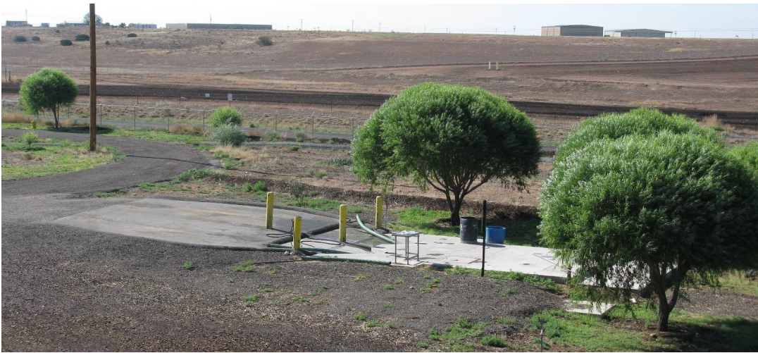
The WWTP accepts Septic Sludge up stream from the treatment plant at its Septic Receiving Station.
