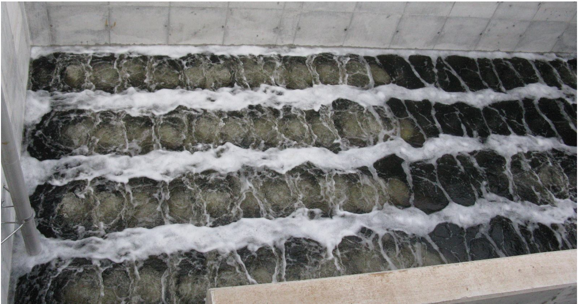
Re-aeration. In the Post Aeration Basin air is added to meet a 5 mg/l or greater of dissolved oxygen at the effluent outfall before being discharged from the Wastewater Treatment Facility.
